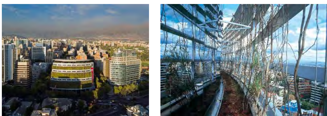
Fig. 4.3.0 Exterior views of the project and inside view showing typical planter at various levels
