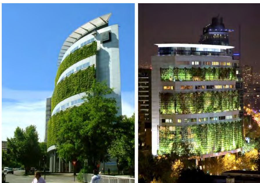
External views of 'Consorcio' building in day and night time
