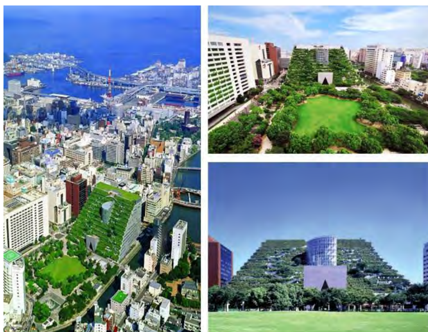
External Views of ACROS Fukuoka Prefectural International Hall
