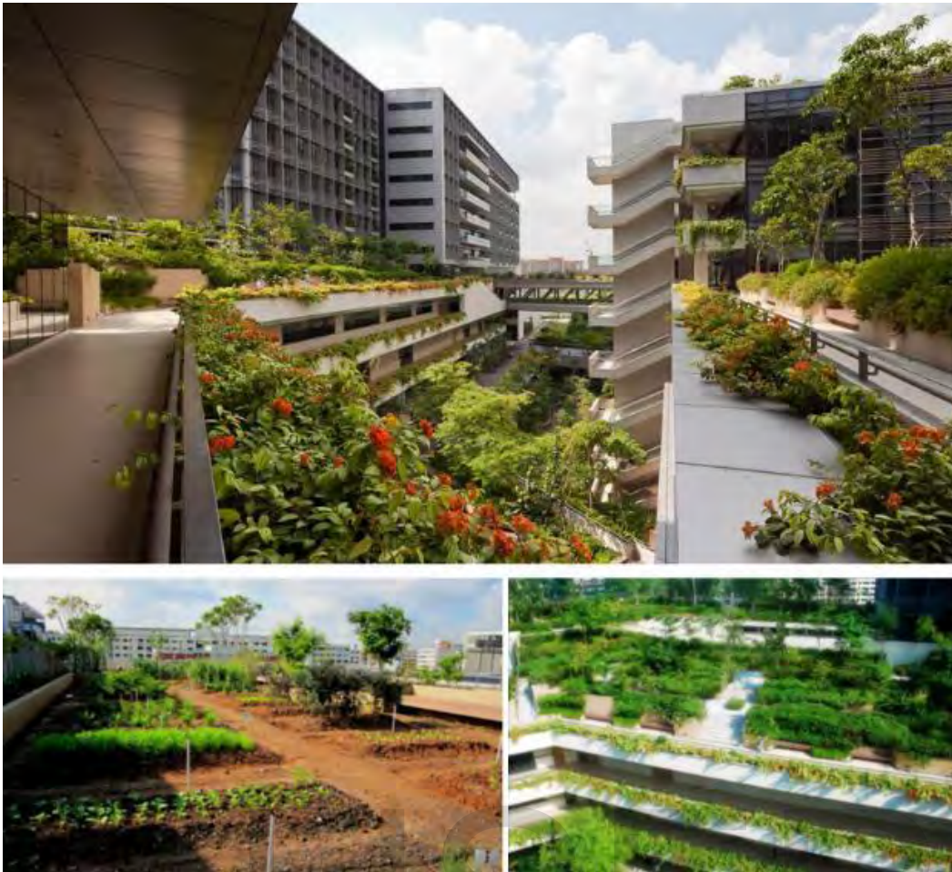
Fig. 4.4.5 Different views of Roof garden and Terrace planters
